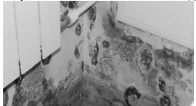
**Fig-2.** Mold and fungus on the inner surface of the damp outer wall
