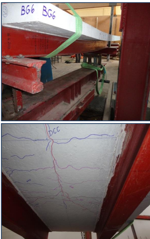
FIG.(7) Crack Patterns at Failure for BG6
