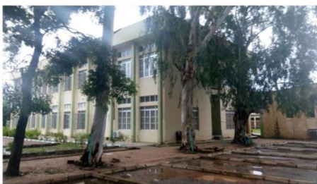
Figure 1.7 showing natural shading at the east elevation Source: Physical Survey
