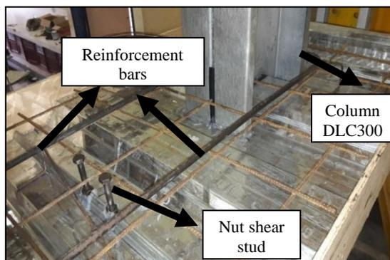
**Figure 4 The rebar and shear connector**
