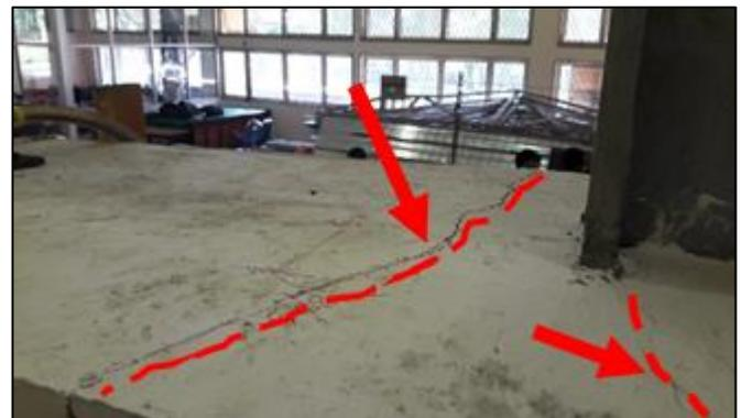
Figure 10 Crack pattern of the concrete slab
