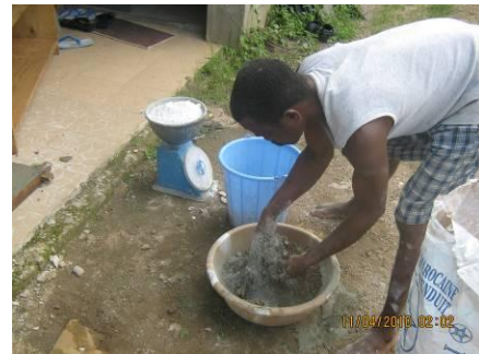
Plate 4: The cement and sand are mixed with water first before adding gypsum.
