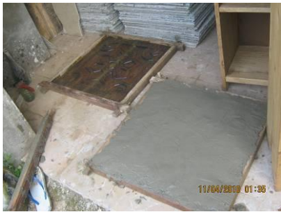
Plate 6b: ( 1\frac{1}{2} sand + 1 cement + \frac{1}{2} pop) mix mould being cast (600 mm x 600 mm).
