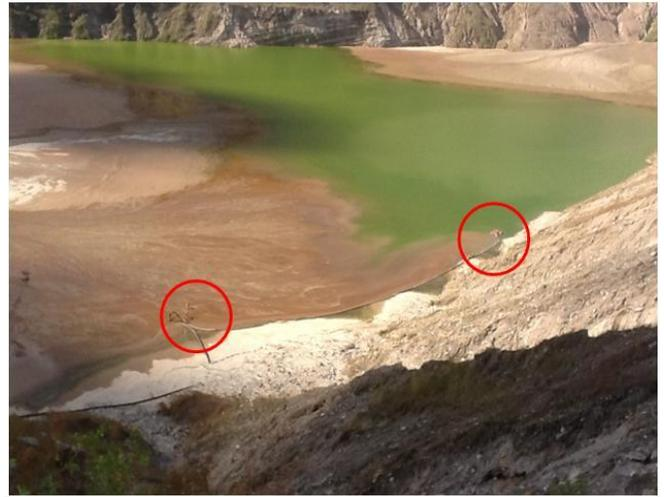
**Fig. 11:** NOP western sump pumping, showing barge and pipelines for underground pumping
