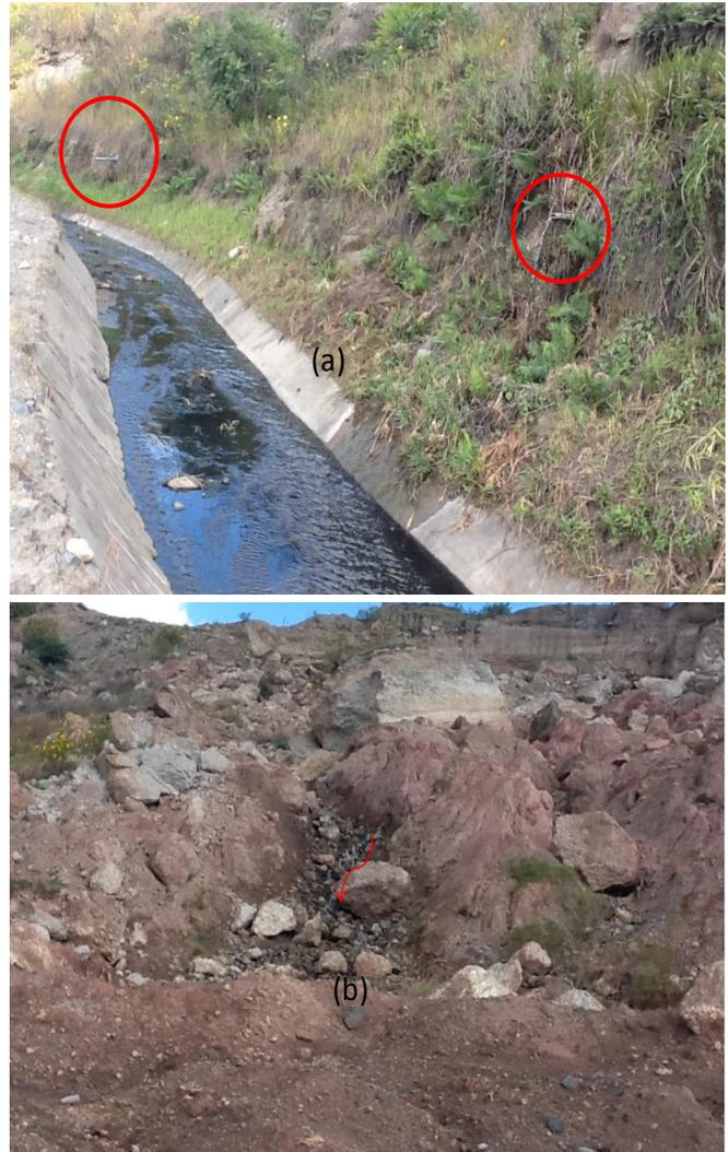
**Fig. 8:** (a) Sub-horizontal borehole geo-drains at NOP with water coming out even after 14 years (b) Subsurface water coming out of the slopes at NOP (arrowed)
