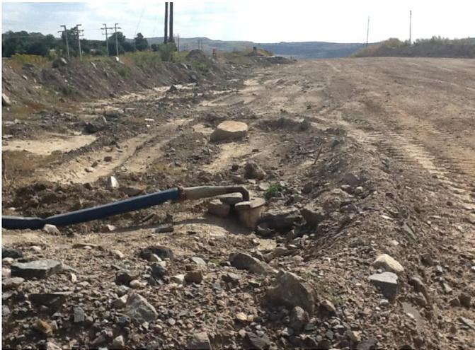
**Fig. 9:** Pumping from perimeter boreholes at NOP and COP D&F
