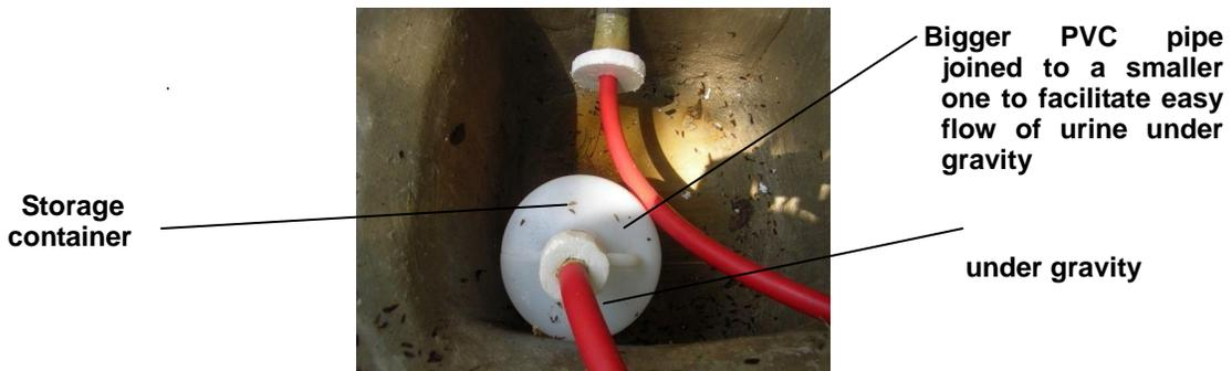
Plate 4. PVC pipe draining urine into an 8 litre container
